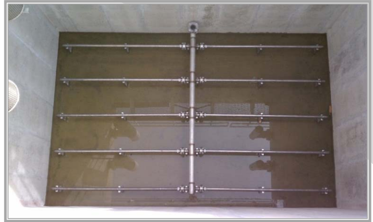
Stainless Steel Aeration Grid Installation
